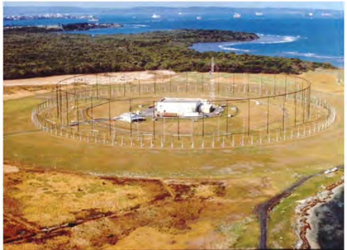
#48. Typical antenna array (AN/FRD-10) of the "Classic Bullseye" program operated by the Naval Security Group for High Frequency Direction Finding (HFDF). (The operations building is shown in the center.) During the Cuban Missile Crisis Bullseye was used to track Foxtrot submarines unbeknownst to the Soviets. (Image source: Wikipedia citing Mark a Dorner - Own work, CC BY-SA 3.0, https://commons.wikimedia.org/w/index.php?curid=27948611 .)
