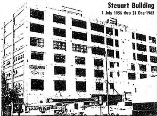
The Stewart Motor Car Company Building, 5 th Street and New York Ave., NW, Washington, D.C. was NPIC's first home. NPIC occupied the top four floors. (Source: McCone History.)
